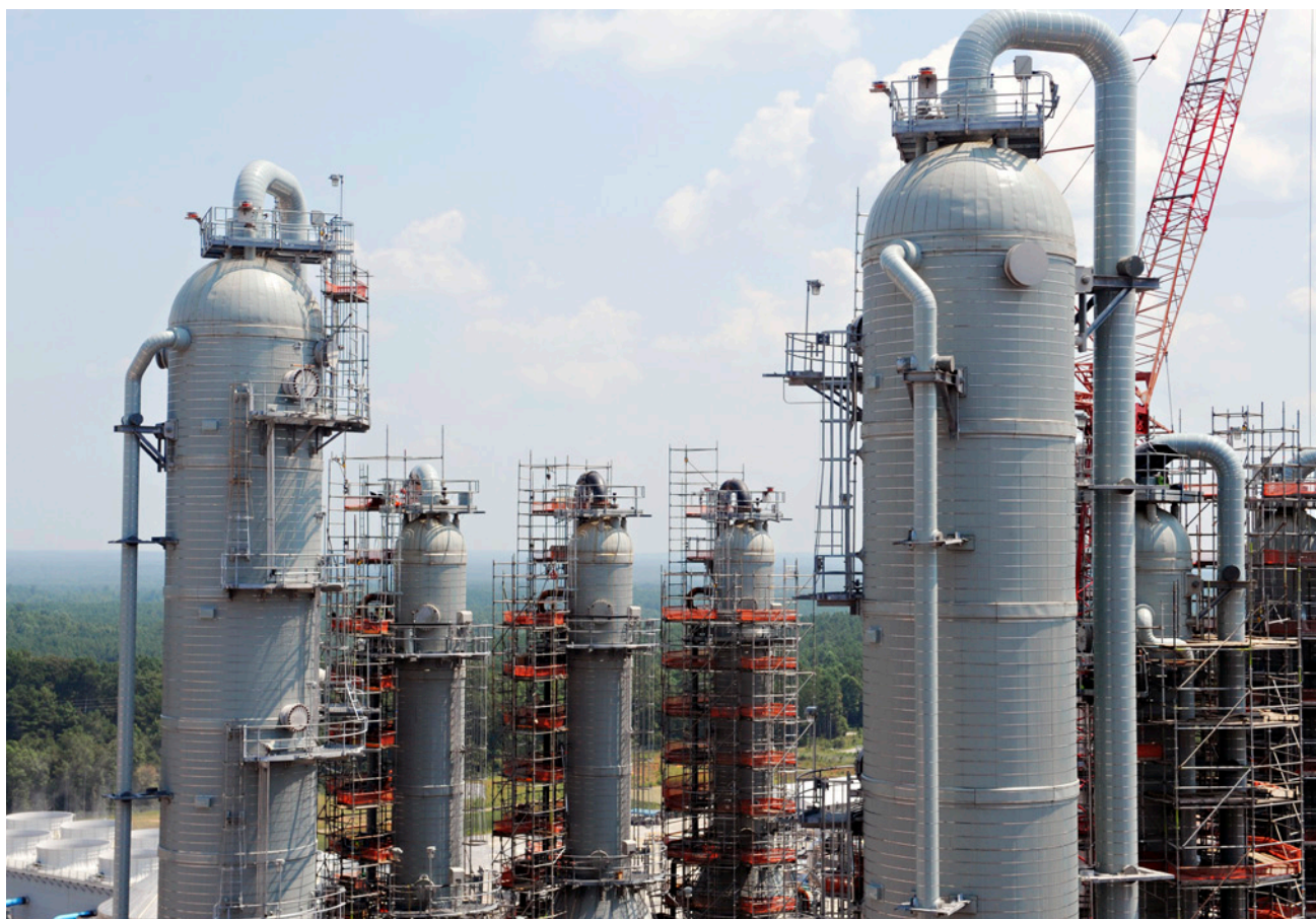
Kemper County IGCC CO 2 absorbers. (Source: Mississippi Power)
