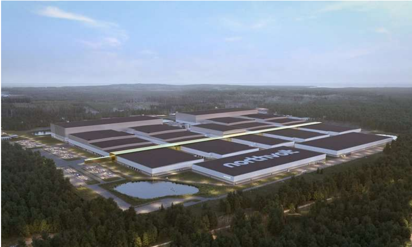
Illustration of the Nothvolt gigafactory in Sweden (under construction)
